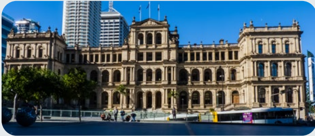
Griffith University CBD Campus Under Construction
