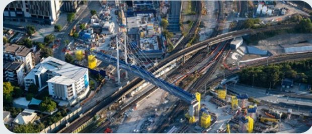
Cross River Rail $6.4 billion – Under Construction
