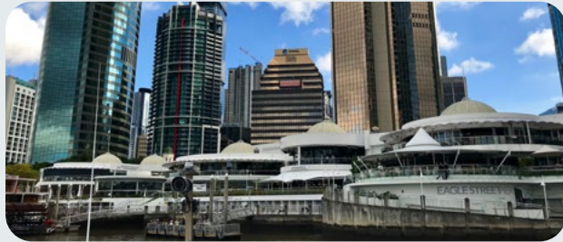
Eagle Street Pier $2.5 billion Under Construction
